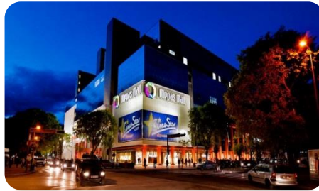
Mepas Mall, Mostar Leasing and development advisory Shopping mall, office spaces and hotel 95,000 m 2 GLA
