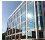
PARKWOOD POINT 13,000-25,353 SF Sublease Jeff Kelley / Russ Jobson
