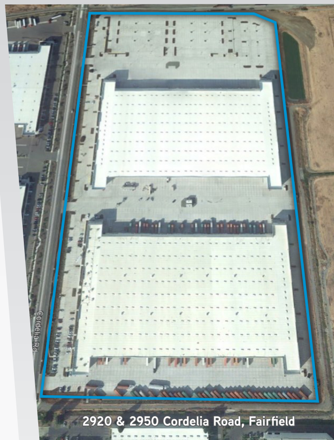
In the largest sale of the quarter, Invesco purchased the recently built two-building, 861,000 square foot Gateway 80 project at 2920 & 2950 Cordelia Road in Fairfield.
