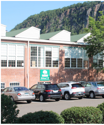
495 Blake Street, New Haven, CT
