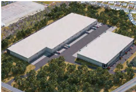
STEELE POINT I & II South 250,750 & 117,000 SF Q4 2017 Delivery
