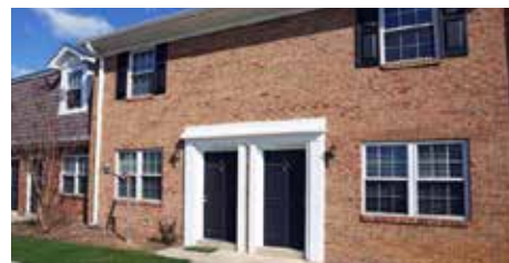
The Arbors Greensboro, NC Units: 150
