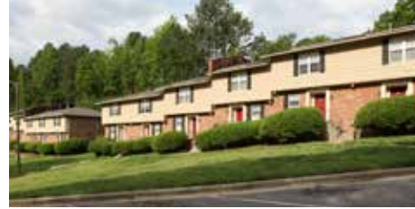
Lantern Square Apartments Raleigh, NC Units: 150
