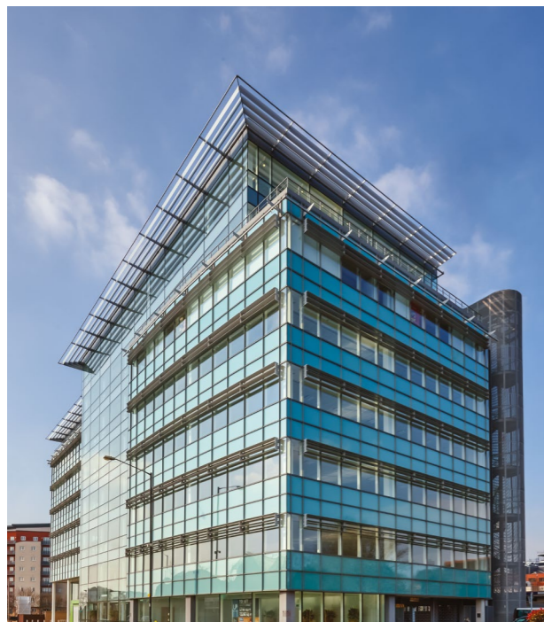
Urban Building, Slough
