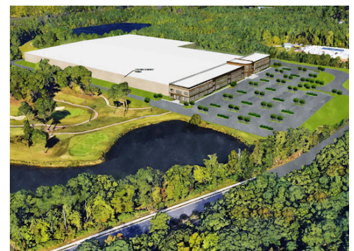
Global Technical Systems (GTS), a Virginia Beach-based provider of advanced engineering solutions for the defense and homeland security industries, is currently constructing a $54.7 million, 500,000-square-foot manufacturing center that would create 1,100 jobs on the former Owl Creek Golf Course in Virginia Beach. Expected delivery is 12/2019.
